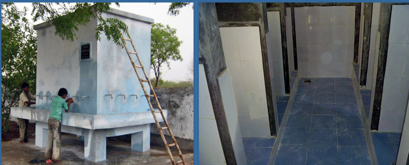
Marian water tank and Sneha toilets
