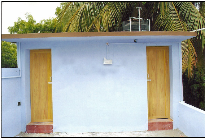
St. Joseph's Home for Children built this new toilet with the funds you provided.
